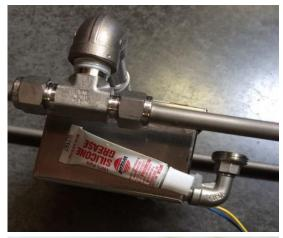
Prior to connecting the Electrical Connection for the Pilot Burner put some Silicon Grease in the connection. A small tube of Silicon Grease came with the SUBEIS system.
