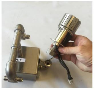
Next, attach the Pilot Burner to the Pilot Burner gas line which is on the side of the box.
