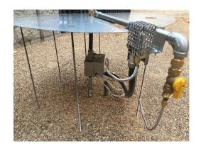
Step 10: Install the Main Burner by threading it onto the Brass Orifice which was installed in Step 7.
