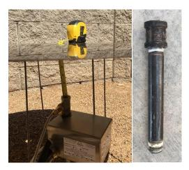
Step 7: Install Brass Orifice in center hole of Flat Burner Pan into coupling described in Step 6 above.
